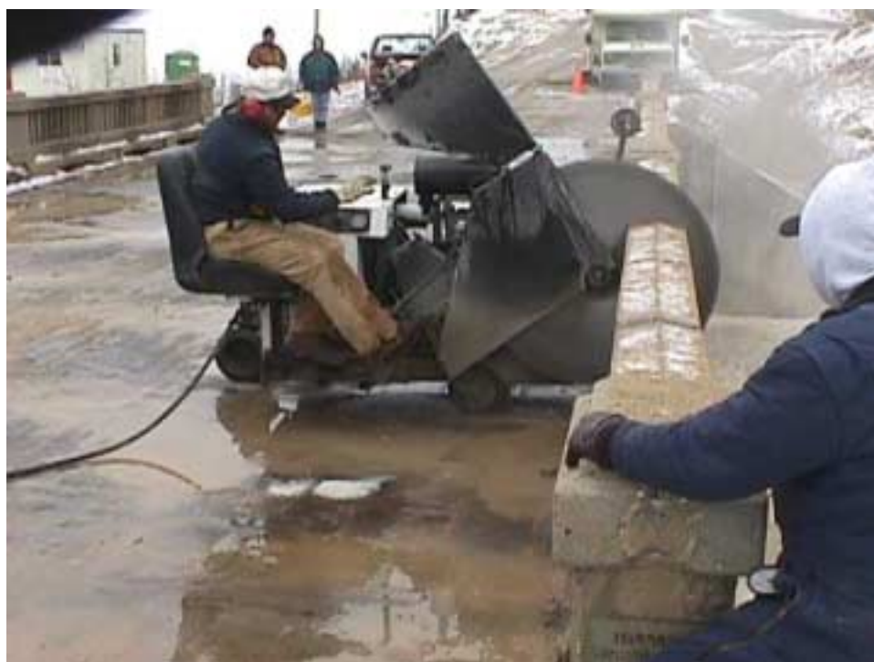
Figure 4.16. Cutting bridge parapet walls.
