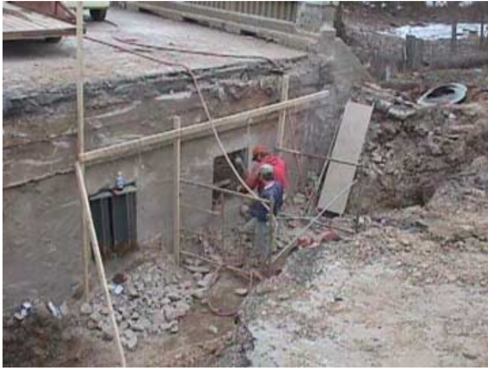
Figure 4.11. Bridge abutment after excavation and cutting.
