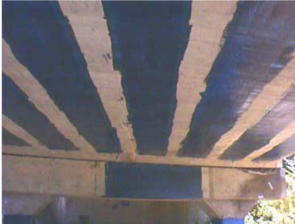
Figure 3.10. Deck 2 after strengthening with CFRP sheets.
