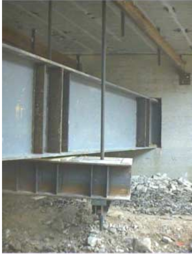
Figure 4.13. Assembled test setup for an end deck.
