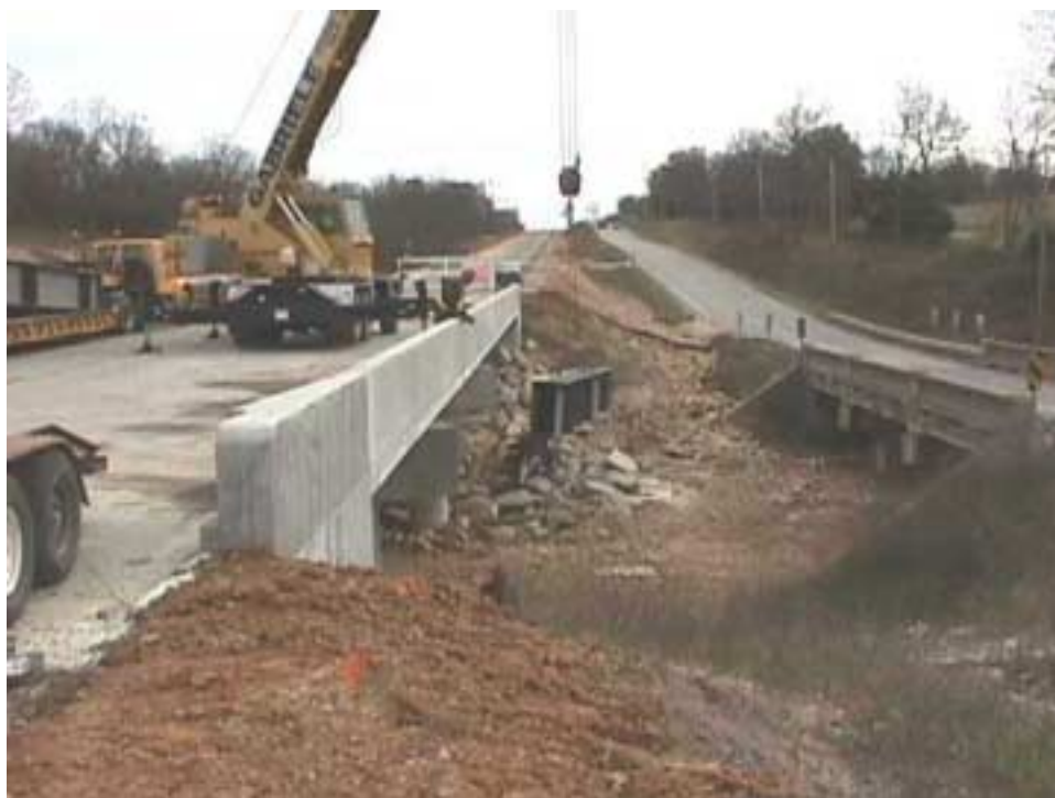
Figure 4.8. Unloading the test setup components at the bridge site.
