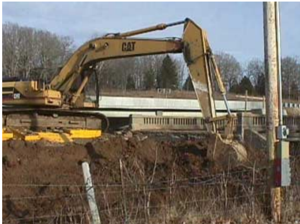
Figure 4.10. Excavating behind the bridge abutment.
