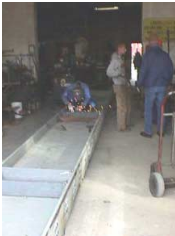
Figure 4.7. Manufacturing the steel girders.
