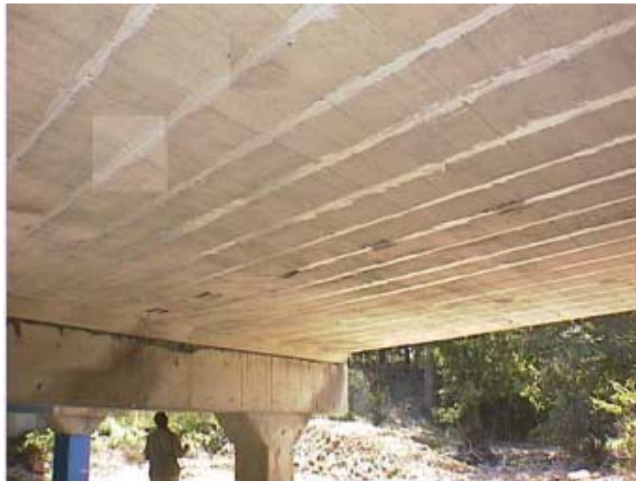
Figure 3.8. Deck 1 after strengthening with NSM rods.
