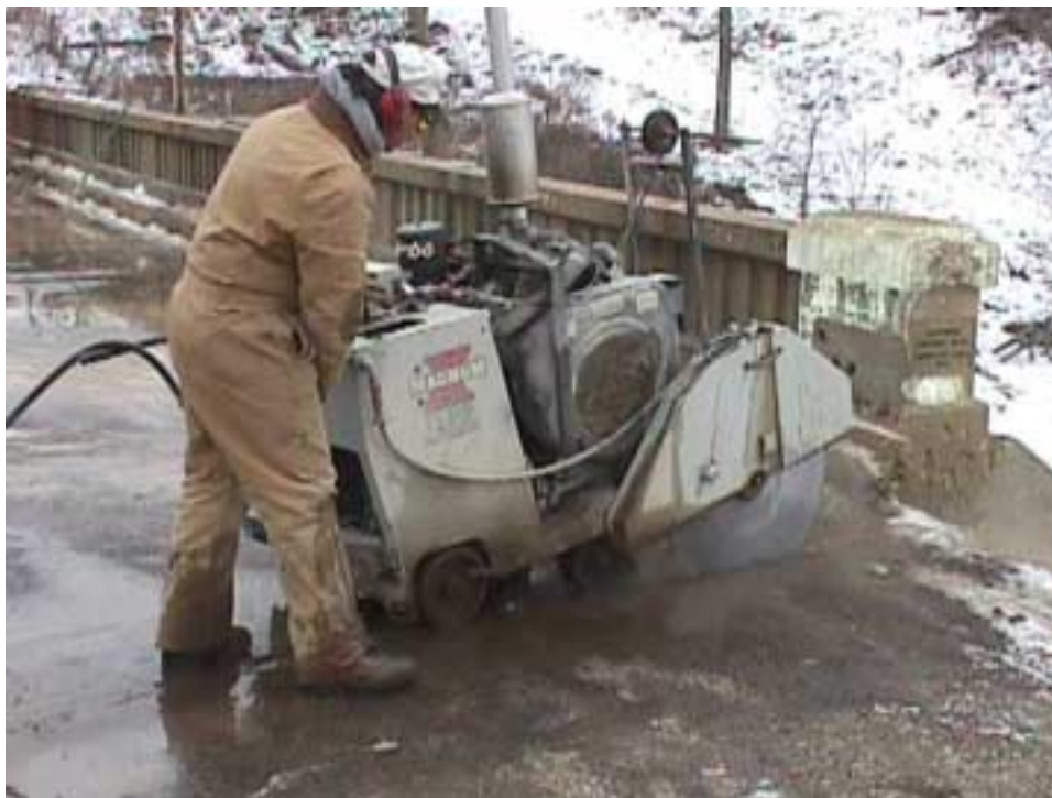
Figure 4.15. Cutting bridge deck joints.
