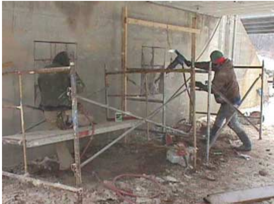
Figure 4.9. Cutting the bridge abutment.
