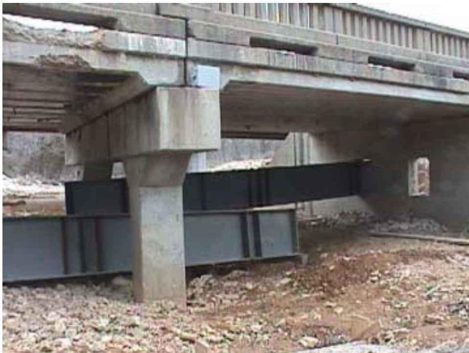
Figure 4.12. Installation of the steel girders.
