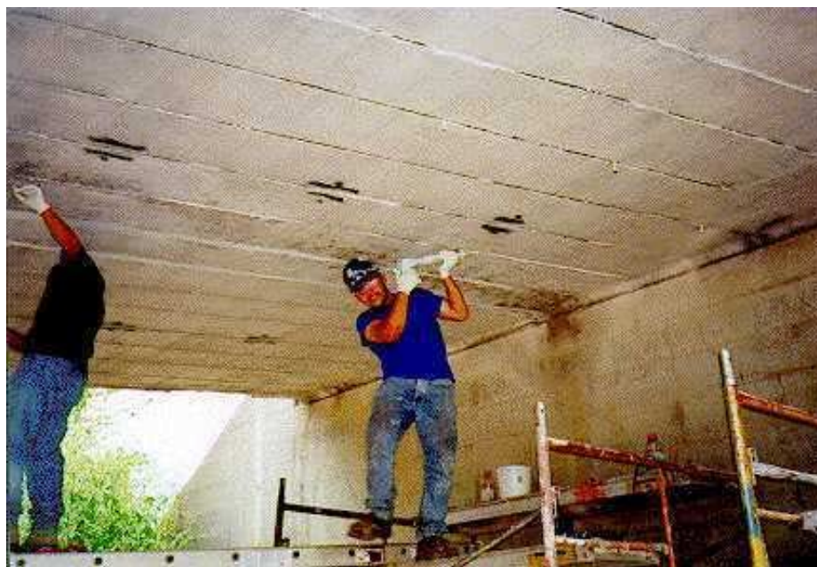
Figure 3.6. Filling the groove with epoxy paste after installing the CFRP rods.
