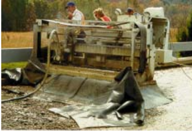
Figure 1: Hydro machine in action. (Note the rubble in front, compared to the milled deck behind.)
