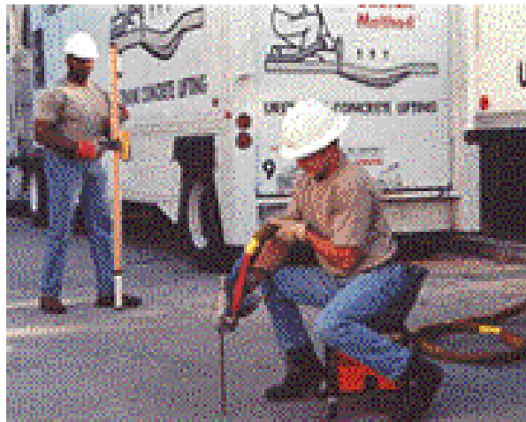
Polyurethane undersealing
