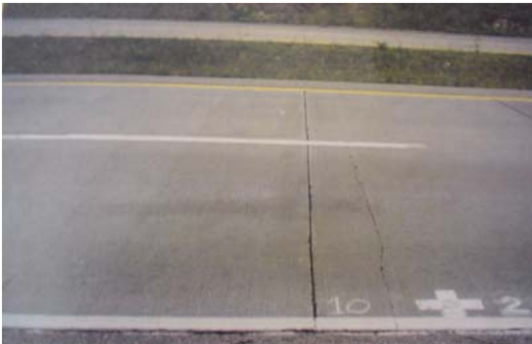
Bonded concrete overlay on NB US 67 in Jefferson County
