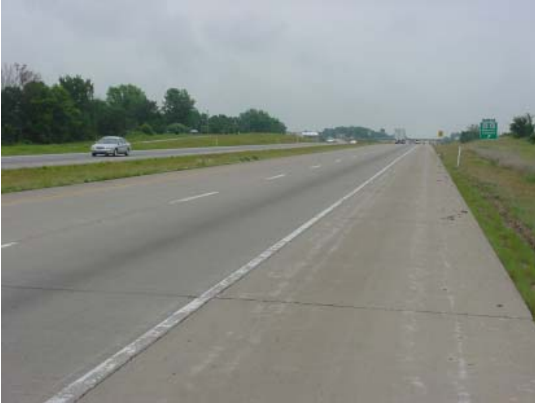
Unbonded PCC on I-70 in Callaway County
