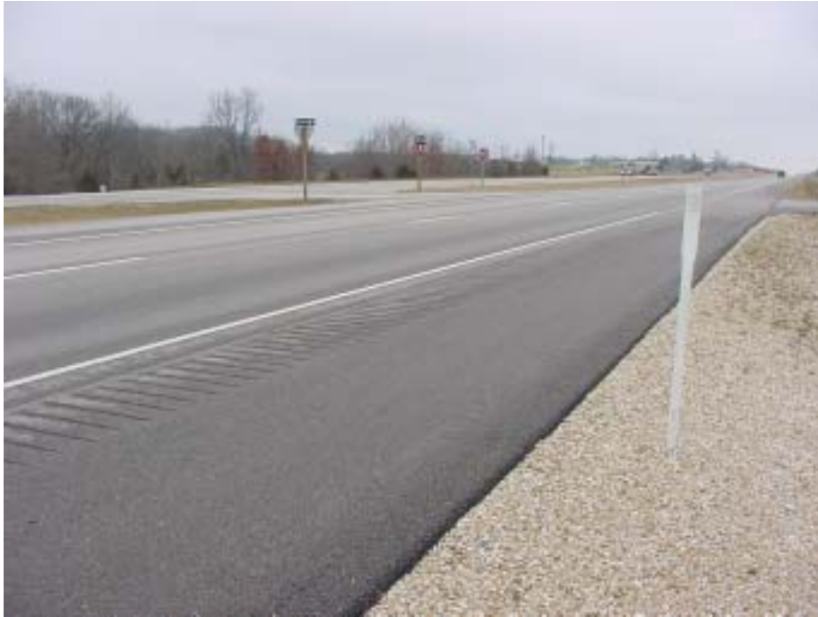
Full depth Superpave pavement on northbound US 63 in Boone County
