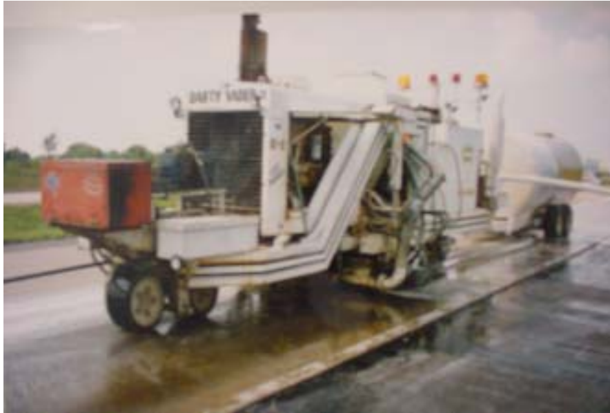
Diamond grinding on I-44 in Greene County
