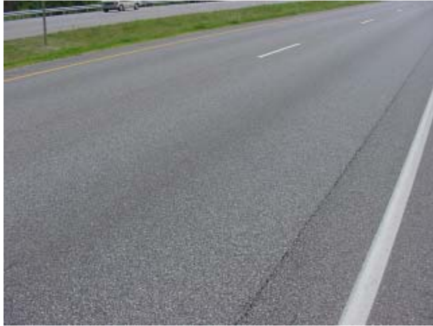
Full depth Superpave AC on US 54 near Camdenton
