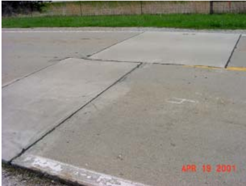
Full-depth repairs
