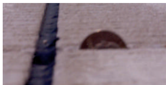
Figure 9. Joint Filler Installed in Longitudinal Joint Figure 10. Quarter Showing Depth of Backer Rod Before Sealing
