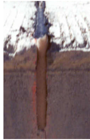
Figure 7. MoDOT Transverse Joint Depth
