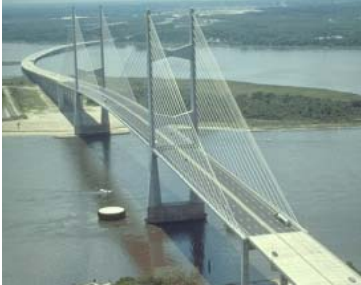
Figure 12: Dames Point Bridge.
