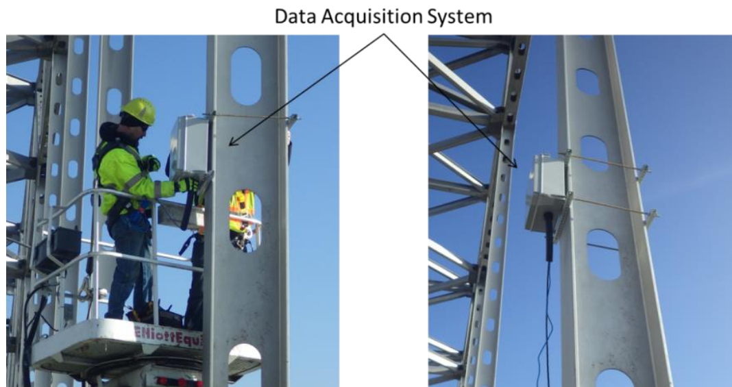
Figure 11. Installation of the data acquisition system on vertical member L22
