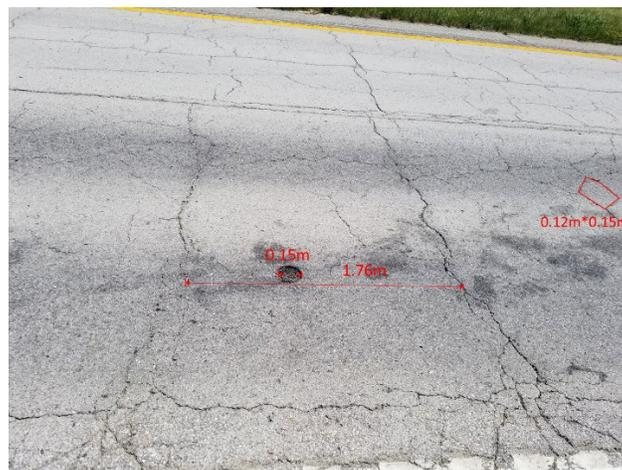
Figure C-1. Block cracks on US63 near La Plata, MO in July 2017, after 9 years of service
