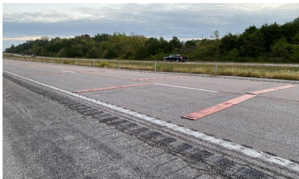
Figure 1: Short-term temporary rumble strips installed on US 63 southbound in Ashland
