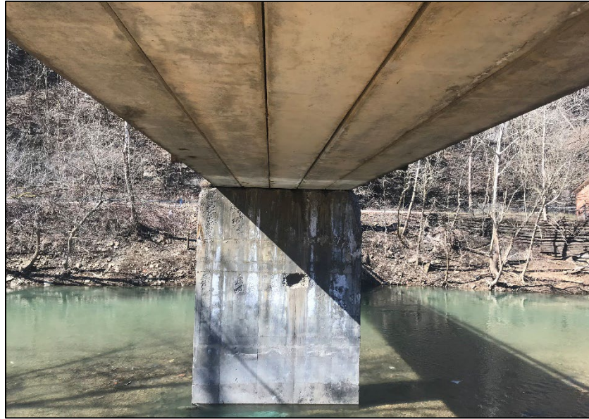
Figure 2. Prestressed concrete box beam bridge with expansion joints suitable for bat use (Photo by Copperhead Consulting).
