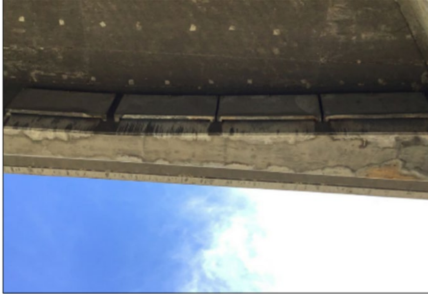
Figure 9. Concrete Oregon wedge style bat habitat with urine staining from Yuma myotis and Mexican free-tailed bats. (Photo used with permission from H.T. Harvey & Associates and HDR 2021)
