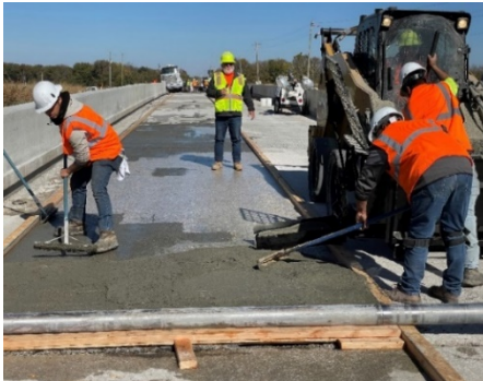
Figure 2: Field implementation of thin-bonded thixotropic UHPC for Route Z Bridge, over Highway 70 in Missouri
