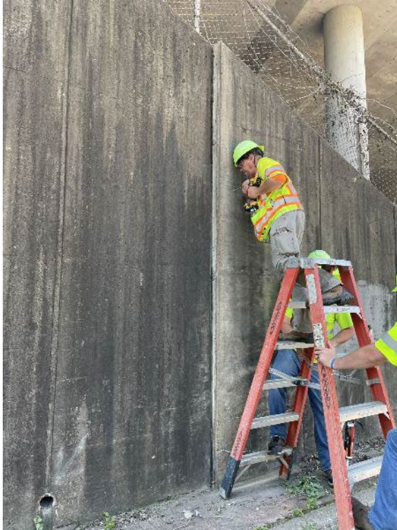
Figure 16. I-44 WB to Berry Road – Tiltmeter Installation
