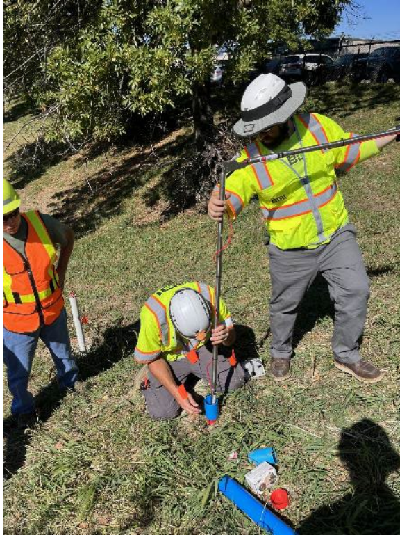
Figure 14. I-44 and Macklind Avenue – Installing In-place Inclinometer
