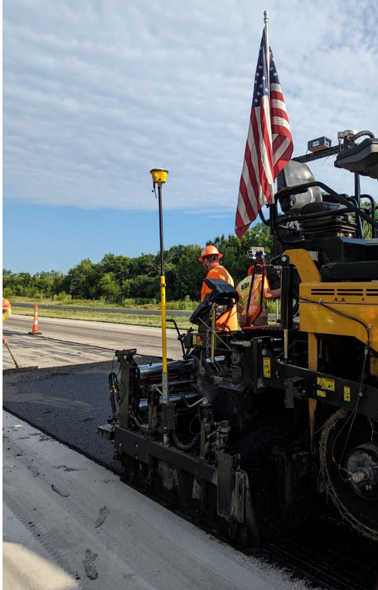
Figure 15. Photo. GPS receiver mounted to paver.
