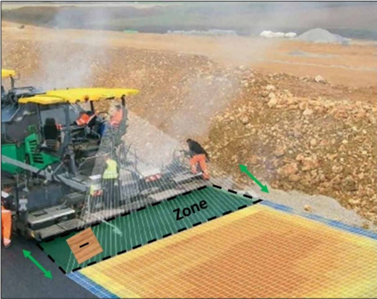
Figure 21. Illustration. Example of placing the event marker directly behind the screed.
