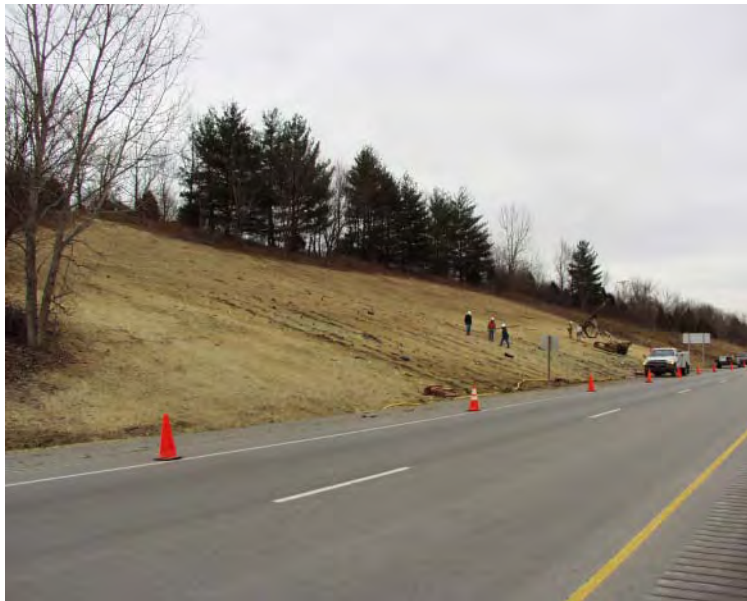
Figure 10.16 Photograph of US54-Fulton test site near the end of installation.
