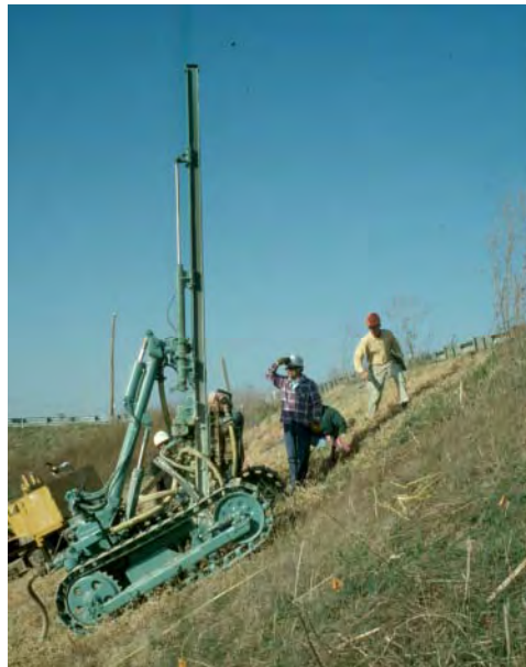
(b) Ingersoll Rand CM150 track-mounted pneumatic rig
