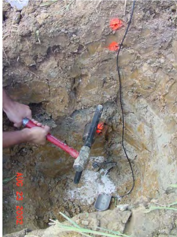
Figure 5.13 Photograph of installation of ThetaProbes ® and Equitensiometers ® in trench.
