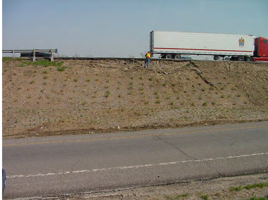
Figure 7.4 Photograph of the I435-Holmes Road site prior to stabilization.
