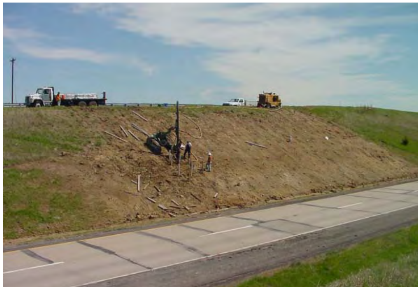
Figure 10.13 Photograph of US36-Stewartsville site nearing the completion of installation.
