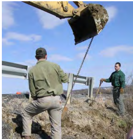
Figure 6.26 Extraction of reinforcing members using backhoe at I70-Emma site
