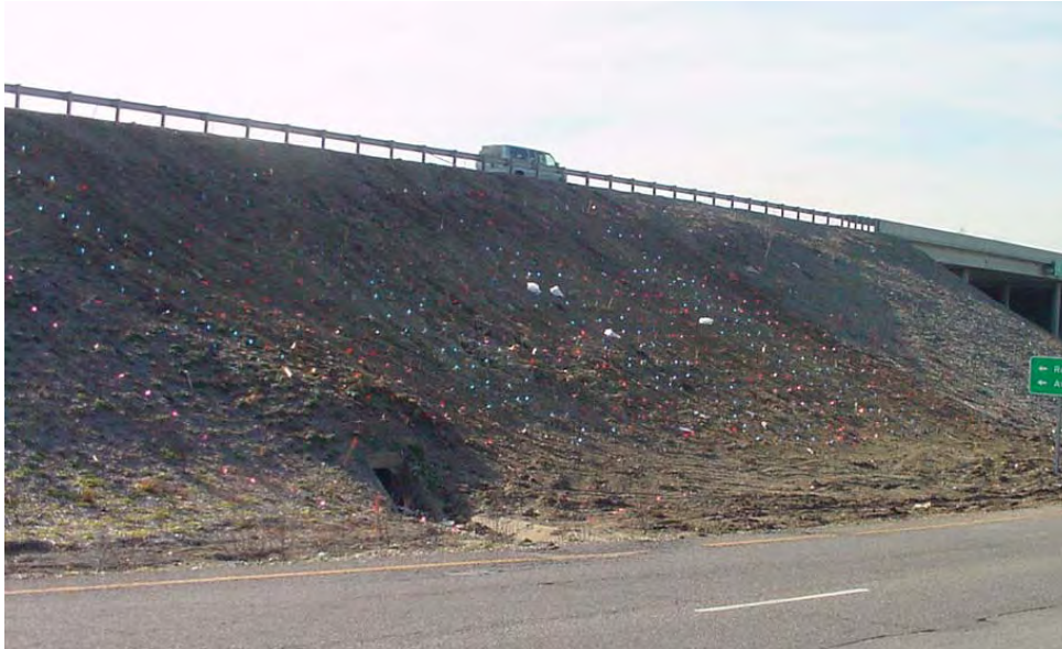
Figure 10.8 Photograph of I435-Wornall Road site following installation.
