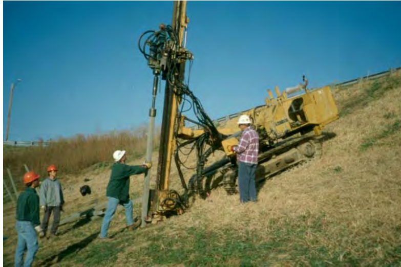
(a) Davey-Kent DK100B track-mounted hydraulic rig
