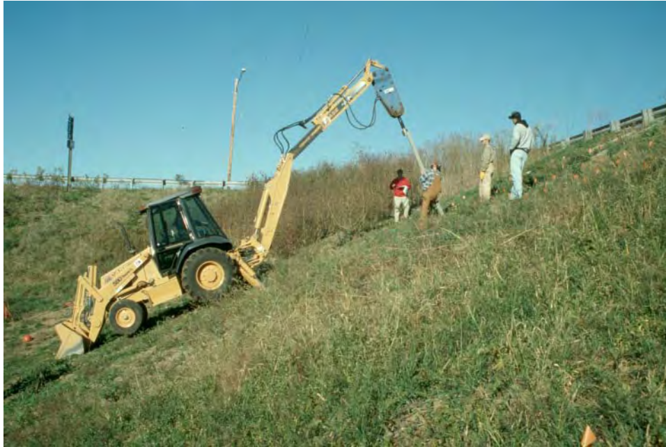
Figure 10.1 Backhoe mounted hammer used for initial installation attempts at the I70-Emma test site during Phase I.
