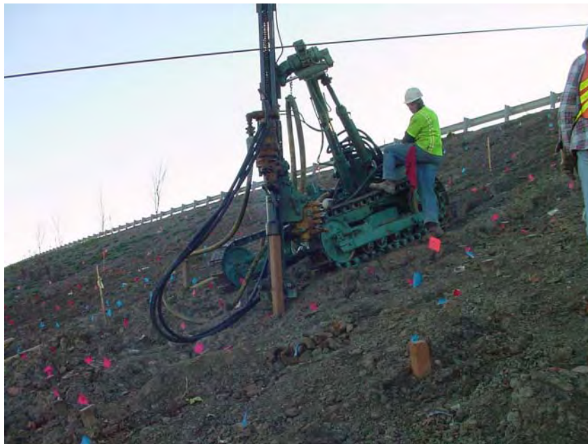
(b) Ingersoll Rand CM150 track-mounted pneumatic rig
