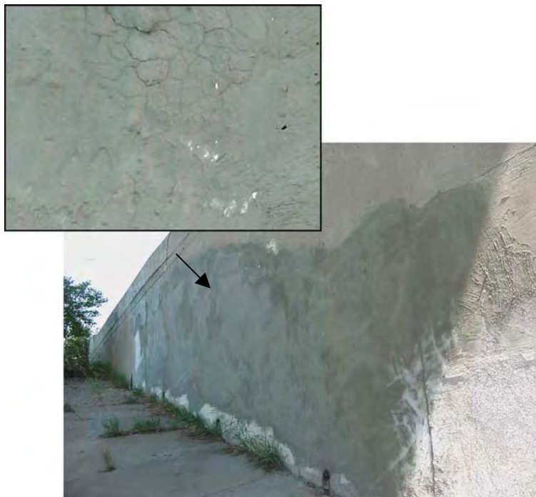
Figure 3 - Bridge A0991 – NW abutment wing wall.
