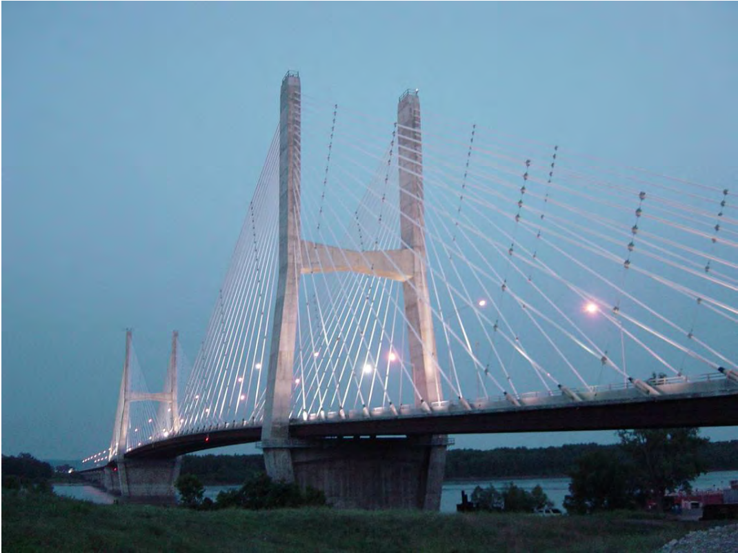
Figure 1.2 Night view of the Bill Emerson Memorial Cable-stayed Bridge
