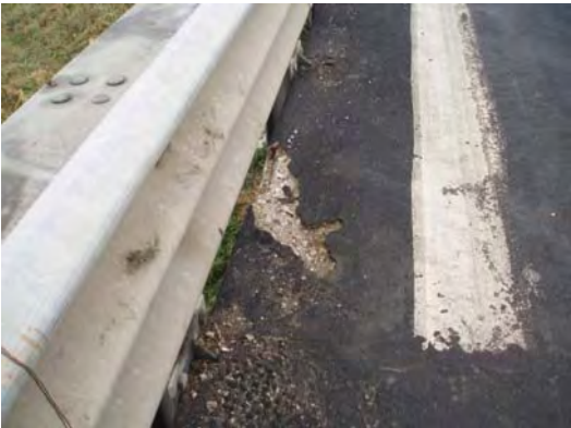
Spalling/loose areas
