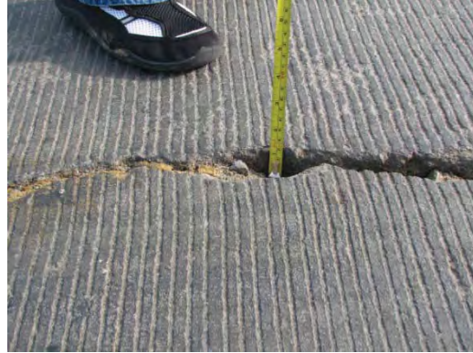
Surface cracking
