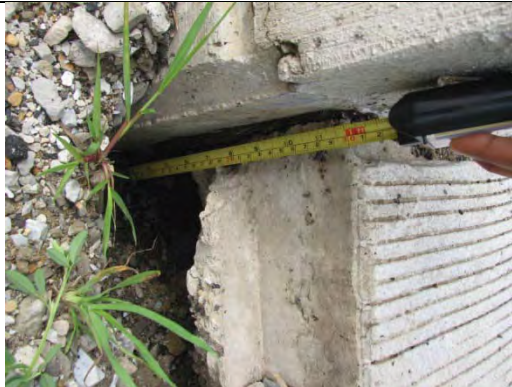
Erosion of soil underneath BAS
