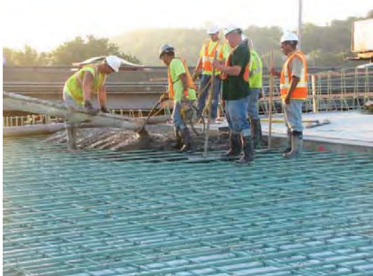
Pouring of Concrete in BAS
