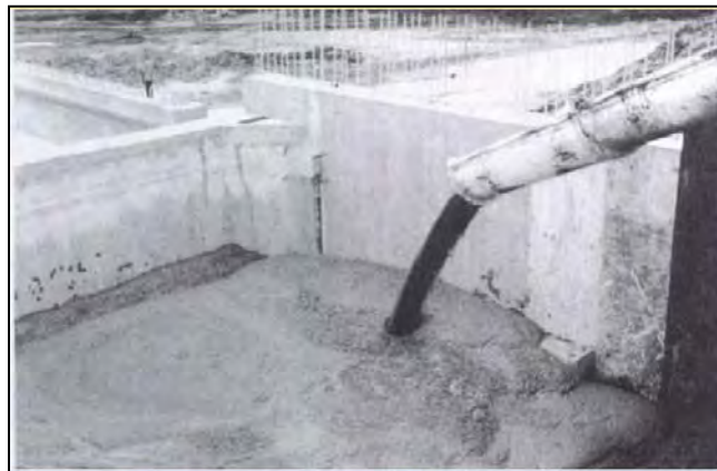
Figure 5-1: Placement of CLSM behind bridge abutment [33]
