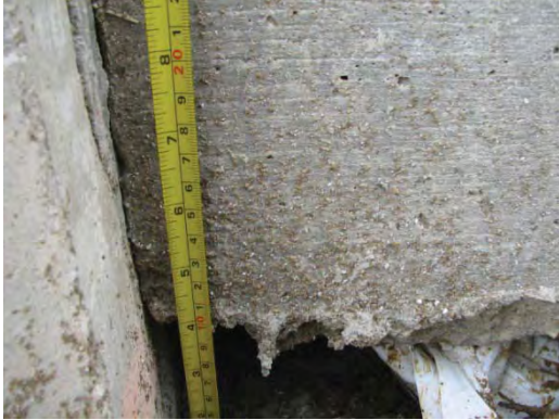
Soil erosion underneath BAS
