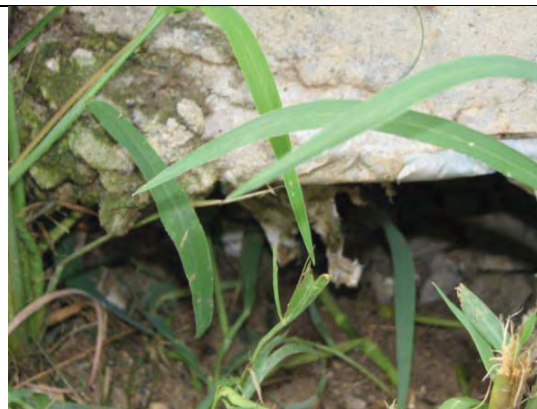
Erosion of soil underneath BAS
