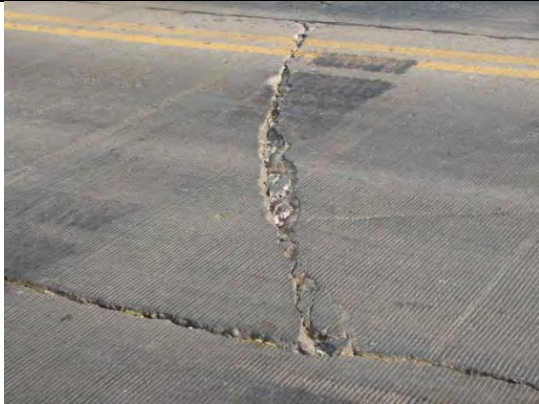
Surface cracking
