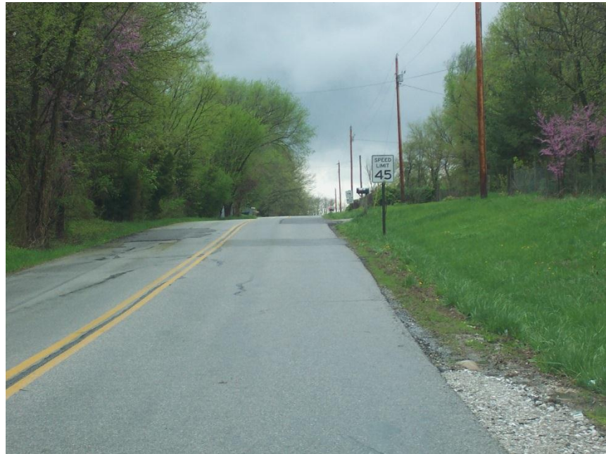
Figure 6.10 Driveway locations difficult to discern due to heavy foliage (Rossy et al., 2009).
