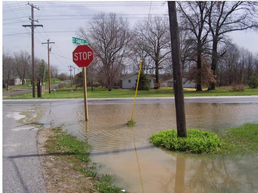
Figure 6.12 Drainage problem at the intersection of St. Charles Road and Route Z (Rossy et al., 2009).
