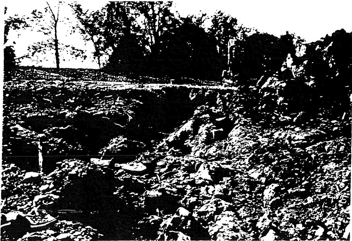
Figure 9: Typical shot muck pile against Williamsons' property line. Pre-split at perimeter just showing.
